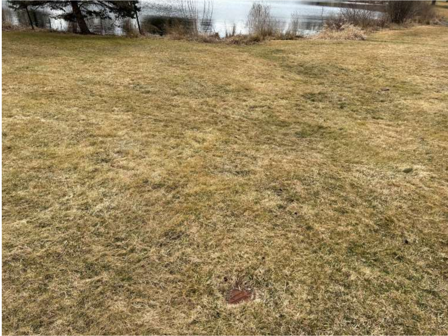
15. Groundwater Monitoring Well #1, Eastern Edge of Pond
