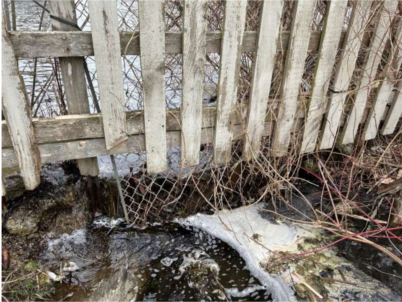
4. Pond Outlet/Weir Structure. Looking North Towards Pond
