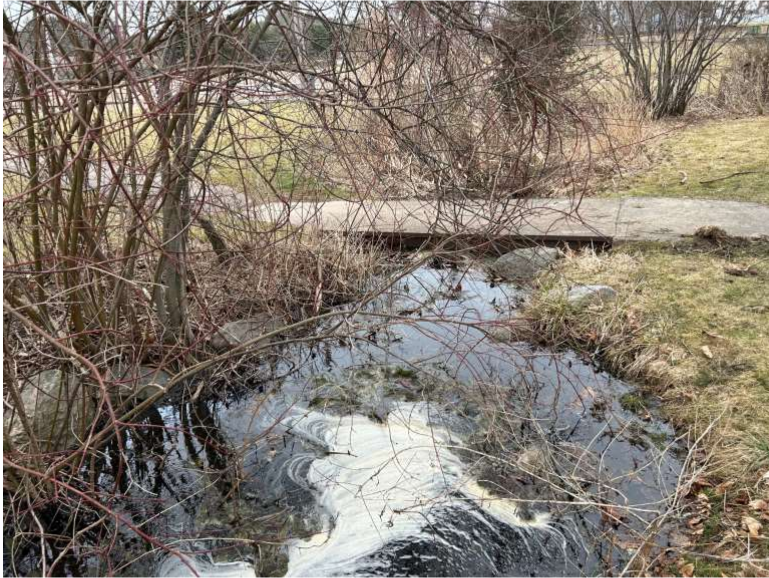
6. Standing at Outlet Looking South Down Swale
