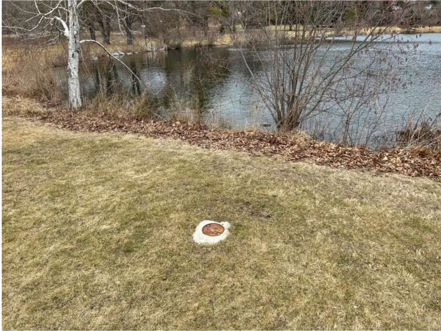
9. Groundwater Monitoring Well #3, Western Edge of Pond
