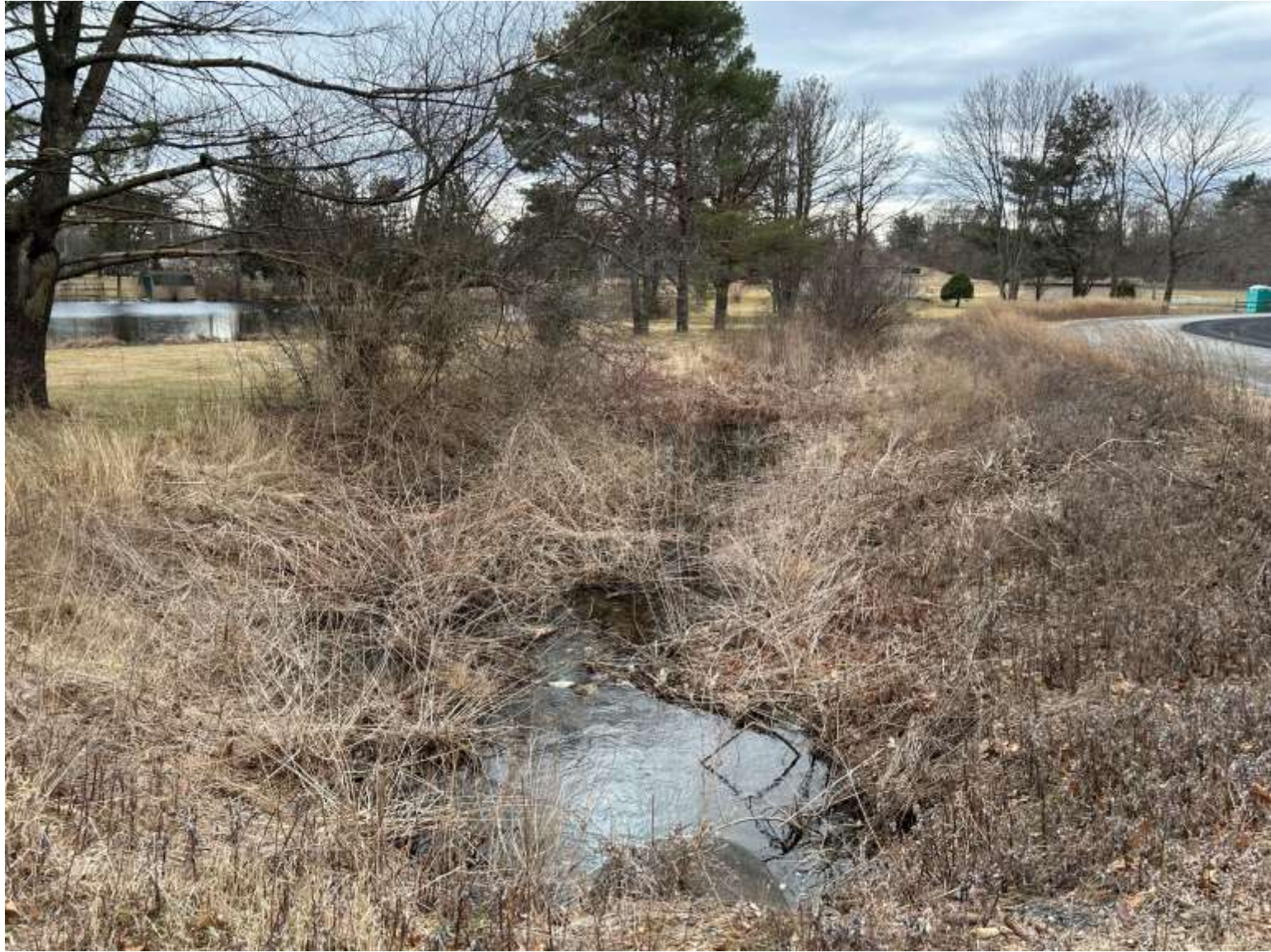
18. Drainage Swale Flowing to Pond & Spigot End of 24" RCP
