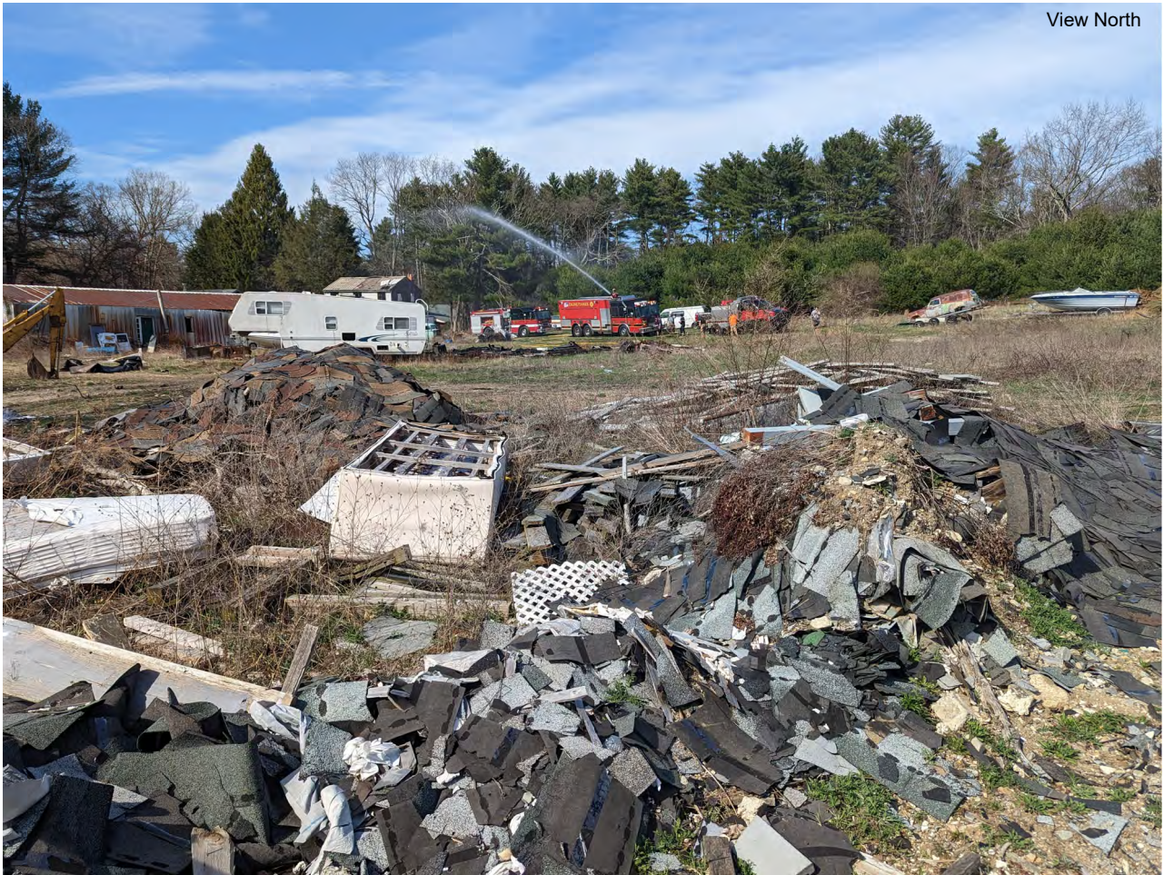
View South - Towards Fall Brook
