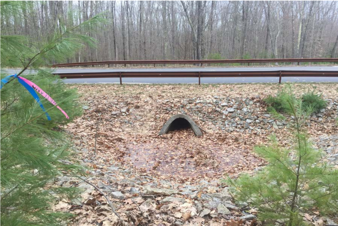
Photo 1: View of Wetland 1 crossing from high school access road looking west.
