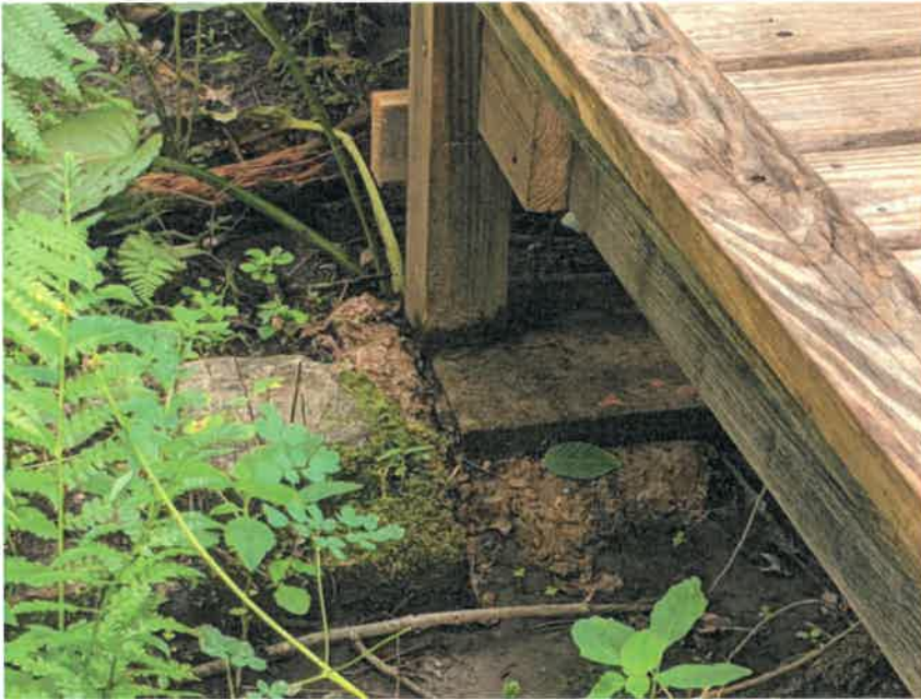
I. Bridge footing shown on cement tile
