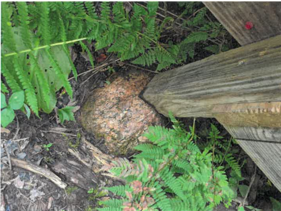
IV. Bridge footing shown on existing rock
