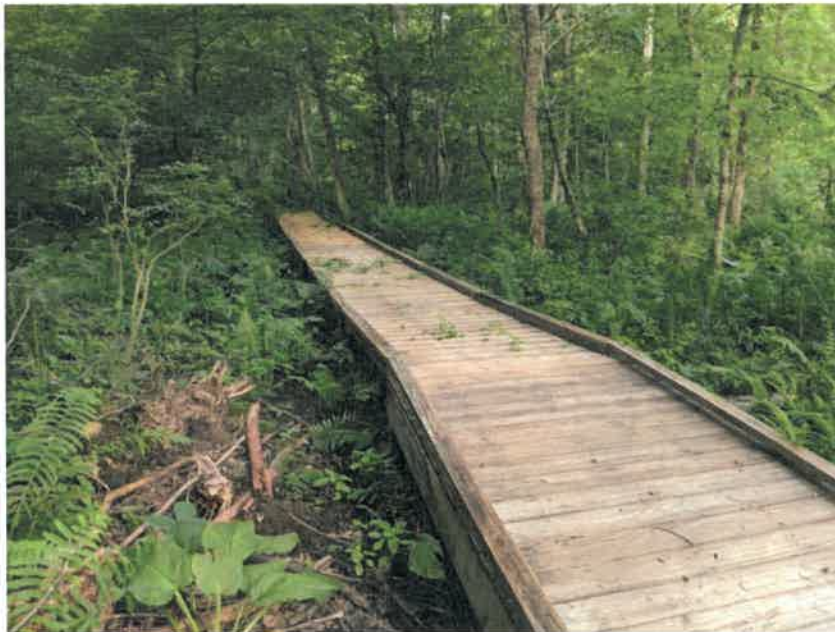
II. Bridge, approximately 4 feet in width, crossing the wetland
