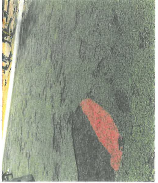
Green area is the original surface top, the orange are the patch work That has been done. As you can see both have deteriorated badly.
