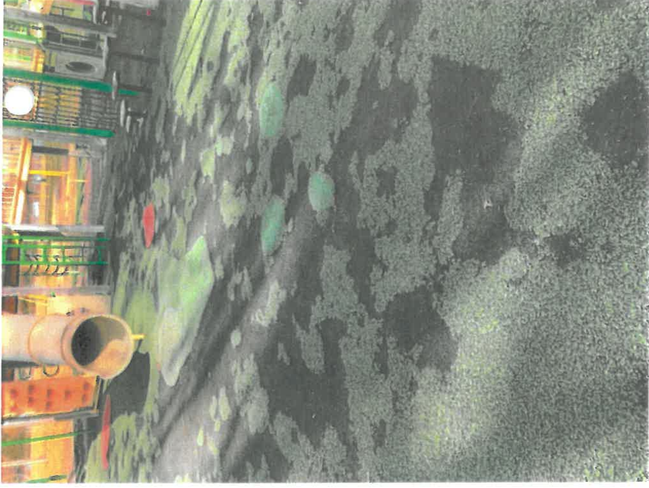
There are some orange and off color green areas that have been patched but as a whole the black area are those that are deteriorated.
