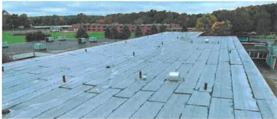
View of the modified bitumen roof system installed above the existing school's north wing (view toward the north). Roof penetrations consist of plumbing vents and roof vents.
