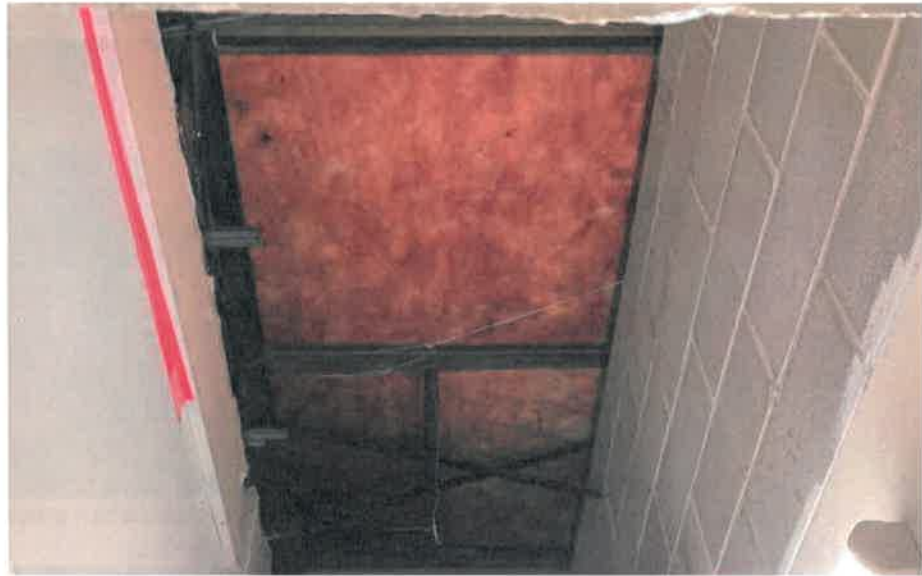
Fiberglass insulation board installed over open-web steel joist framing.
