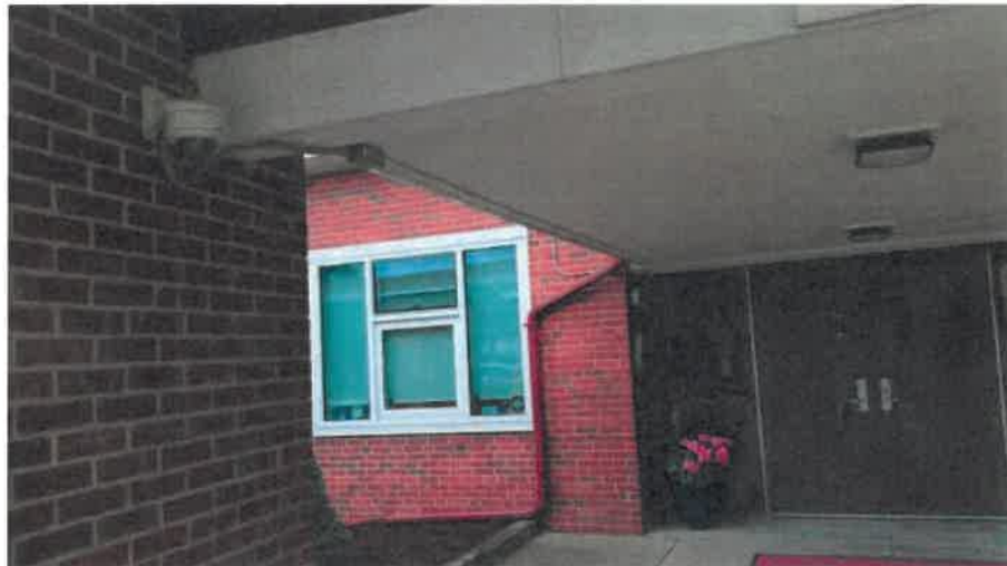
Existing exterior video surveillance cameras at main entry.
