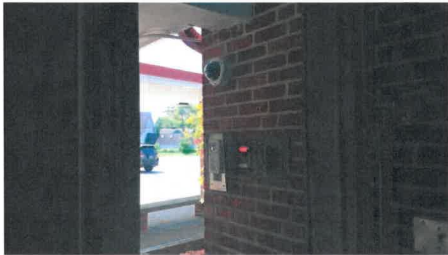
Exterior video intercom entry system.
