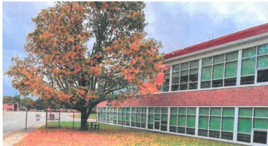
Classrooms typically have expansive window walls spanning the full room width along the exterior wall above radiant heating in millwork enclosures,
