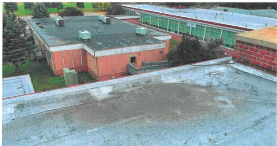
View of the modified bitumen roof system installed above the existing school's north wing (view toward the north). Roof penetrations consist of plumbing vents and roof vents.
