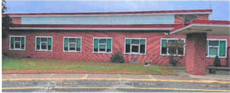
Punched window openings to offices along the main entry level and a view of the translucent panel glazing system at the south side of the Gymnasium – Auditorium, above.
