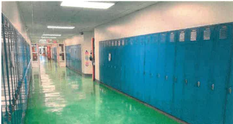
A plaster infill above painted metal lockers located along corridors.
